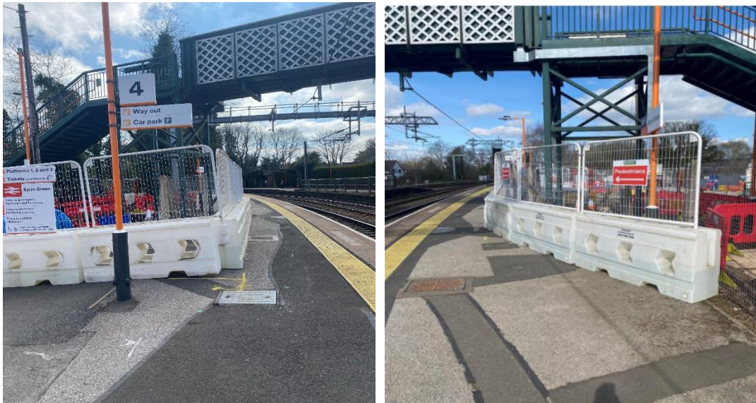
Firey Hill Road closure and installation of traffic management in preparation for platform 1 works
