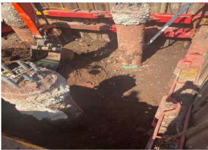
Excavate, install sheet piles and bracing platform 1 lift pit
