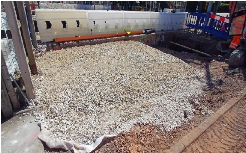
Foundation works for Platform 1 lift motor room
