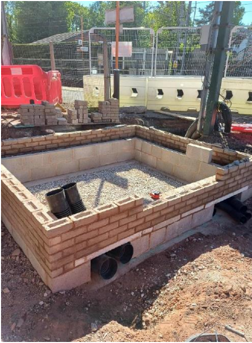
Stone for Piling mat on platform 1
