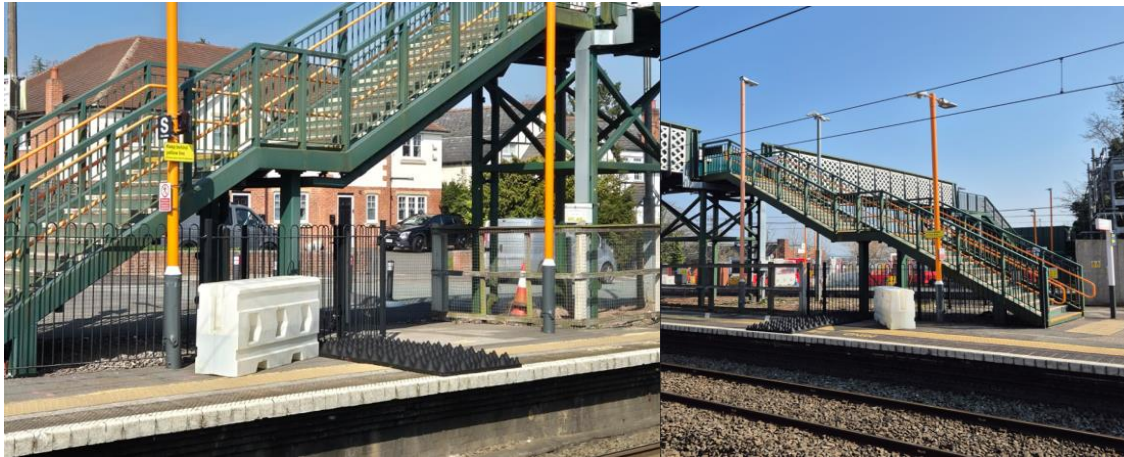
Existing station fencing on platform 4 removed and water filled barriers installed to prepare the working area for the excavation of the lift motor room foundations
